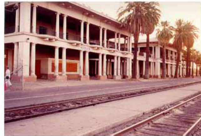
EL GARCES SANTE FE TRAIN STATION AND HARVEY HOUSE
